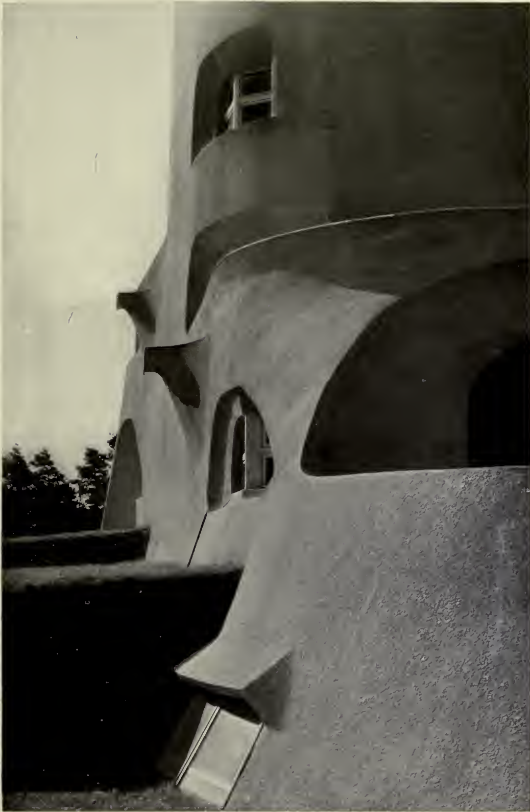
Typical detail of the Einstein Tower showing plastic architecture conceived and executed in reinforced concrete. Potsdam. Erich Mendelsohn, Architect.
